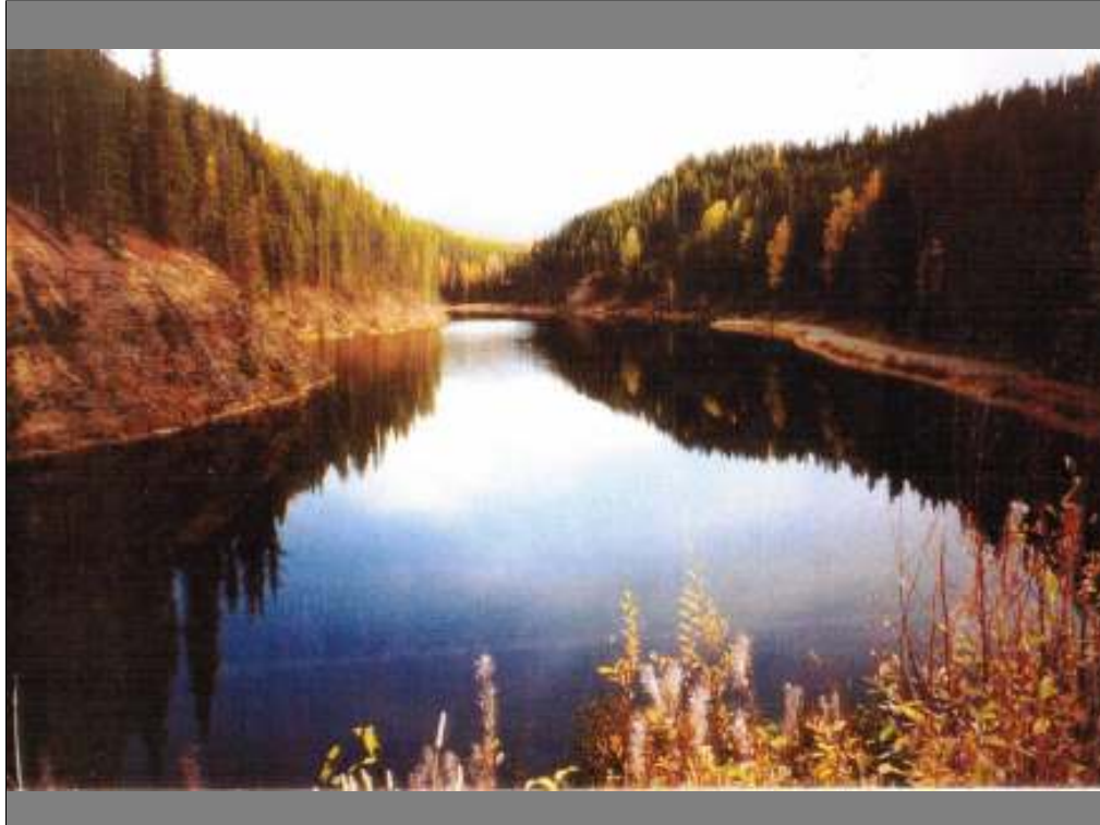
2 The City of Kimberley Water System : Mark Creek reservoir
